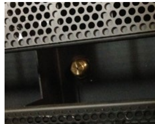
Figure 13.c Removing the orifice
